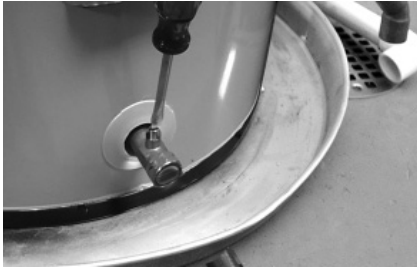
Figure 10 - Draining the old water heater.
