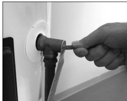
Figure 38 - T&P Relief Valve
