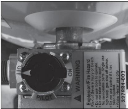
Figure 37 - Turn gas control knob OFF.
