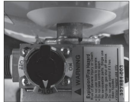
Figure 33 - Gas control/valve top view.
