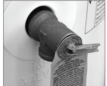
Figure 24 - Temperature and Pressure Relief Valve
