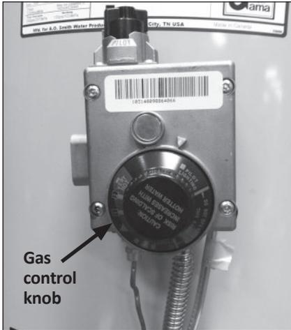
Figure 17 - Turn gas control/temperature knob OFF.
