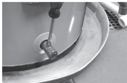
Figure 20 - Draining the old water heater.
