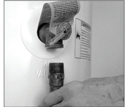
Figure 21 - Removing the T&P Relief Valve discharge pipe.
