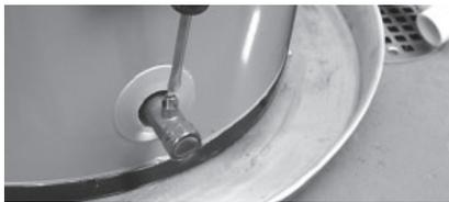
Figure 39 - Draining the water heater.
