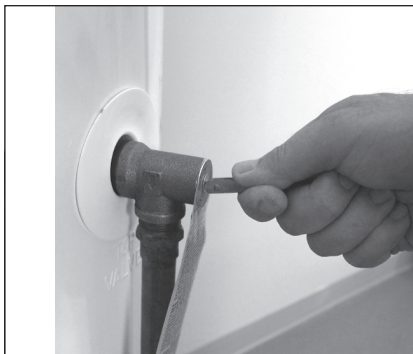
Figure 48 - T&P Relief Valve.
