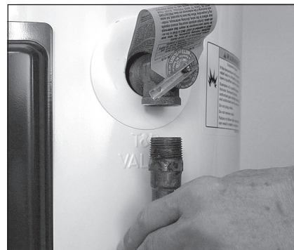
Figure 13 - Removing the T&P Relief Valve discharge pipe.
