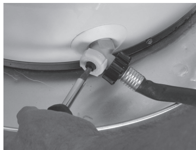
Figure 12 - Draining the old water heater.
