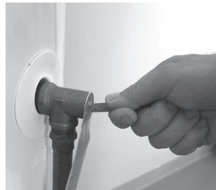
Figure 46 - T&P Relief Valve
