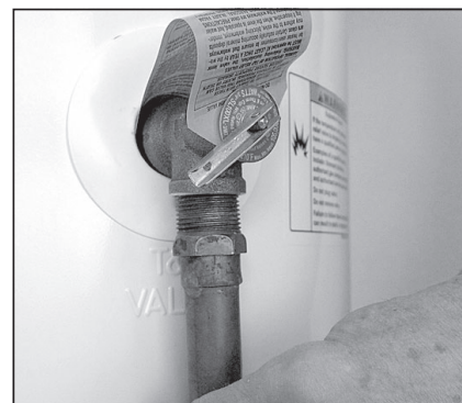
Figure 16 - The T&P Relief Valve discharge pipe must be installed properly and piped to an adequate drain.
